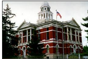
Second County Courthouse Built 1888
